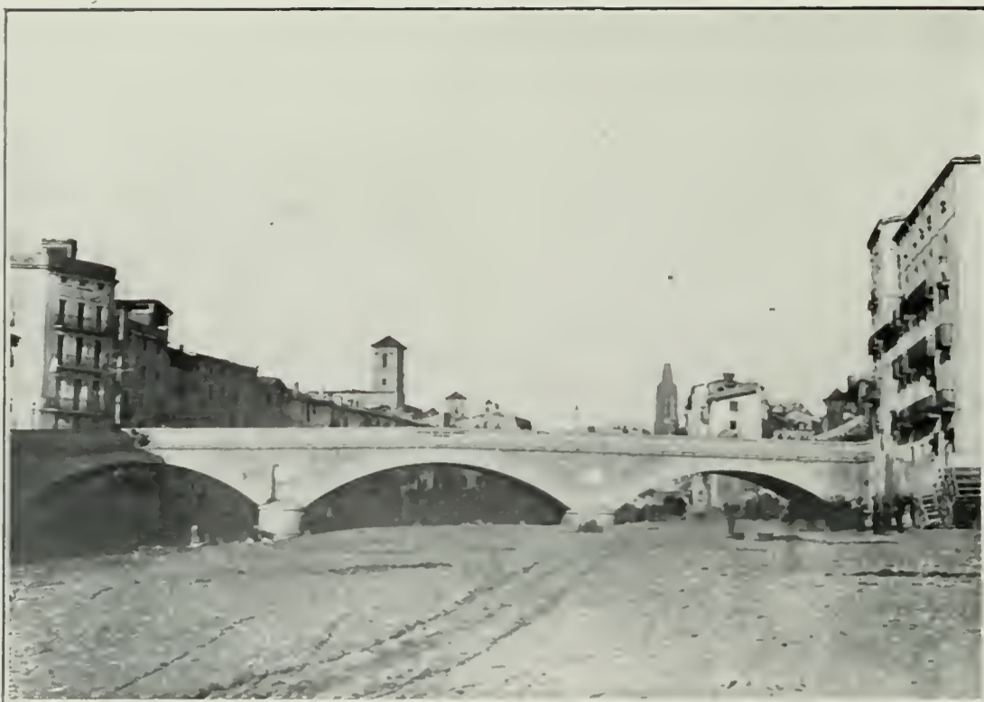
BRIDGE OF ISABEL II., GERONA
